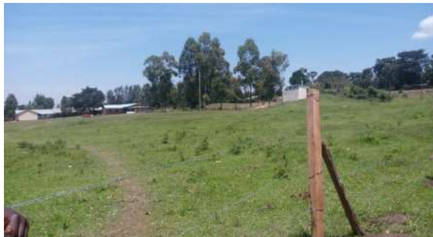
A view of Matumbai primary school. Just constructed fence
