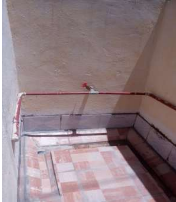
Just completed Urinal for girls at Matumbai primary school
