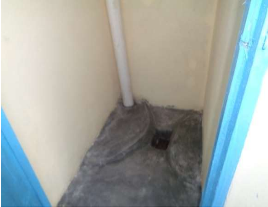
Inside view of a pit latrine
