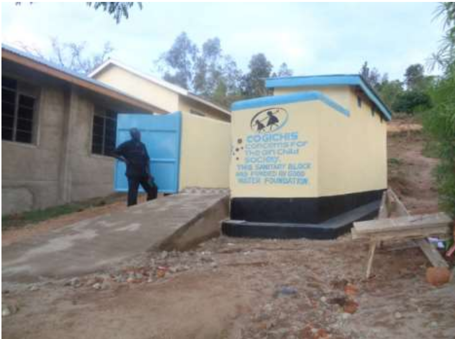
Side view of the sanitary block
