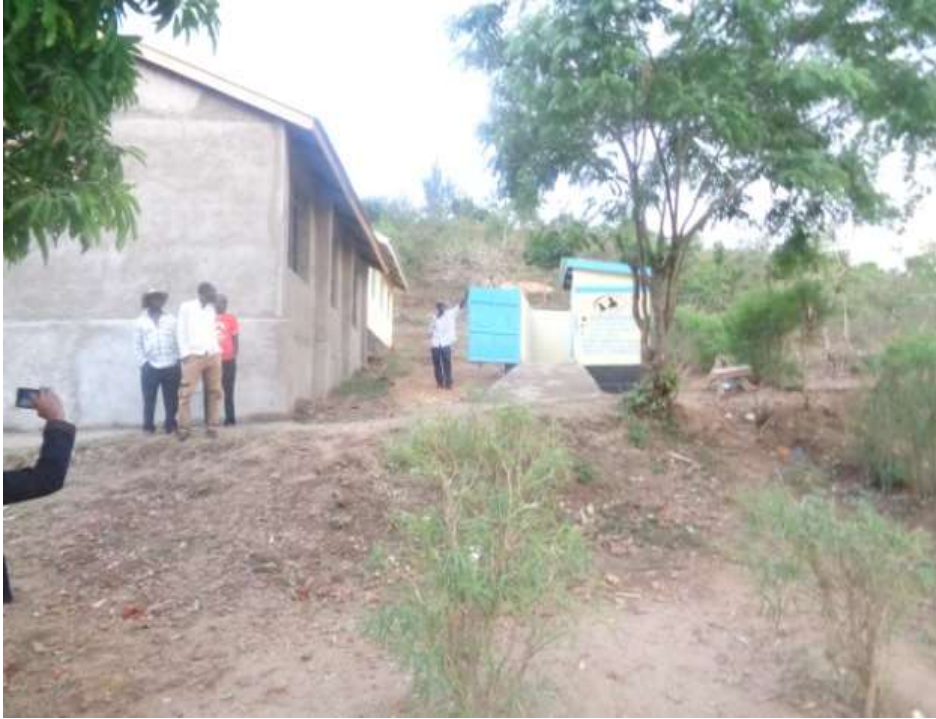
Committee members viewing the finished sanitary block.
